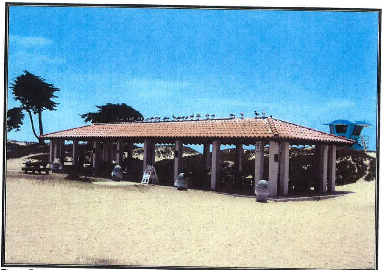
Figure 7. Existing ramada, lying south of the parking lot and adjacent to the dunes, which would be demolished and rebuilt as a new, shade sail structure.
